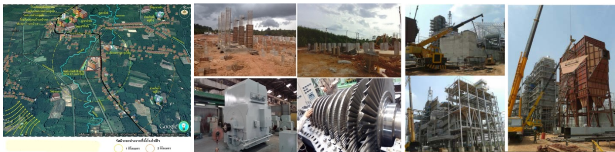
Fig. 2 Overall of Biomass Power Plant Construction in Southern Thailand (Install Capacity 9.5 MW)
